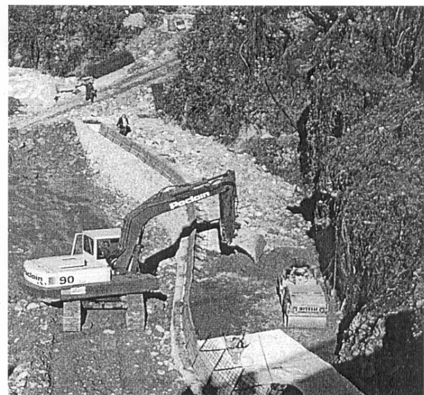
Figure 7. Construction of first layers of reinforced earthfill. In foreground the reinforcing metal braces.
