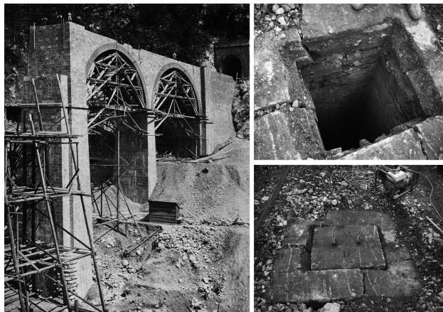
Figure 17. Left, the two southern spans as they were constructed (AA.VV. 2010). Right, the mine shaft discovered inside the central pier.
