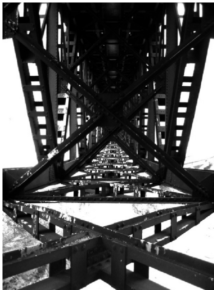
Figure 11. Inside of the truss (the deck is on top). Paintwork on the lower parts of the truss has extensively peeled off, exposing the underlying orange-coloured primer (March 2007).
