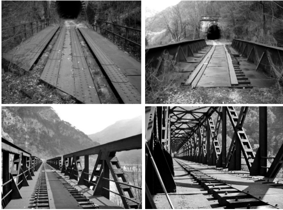
Figure 4. Examples of metallic bridges on the Pontebbana rail line (years 2007-2008). Top left, the small bridge over Rio Confine with twinned girders (on the municipal border between the villages of Dogna and Pontebba). Top right, the bridge on Rio Pontuz with plate girders (Dogna). Bottom left, the pony truss bridge “Ponte Peraria”. Bottom right, the through truss bridge “Ponte della Chiusa” (Chiusaforte).
