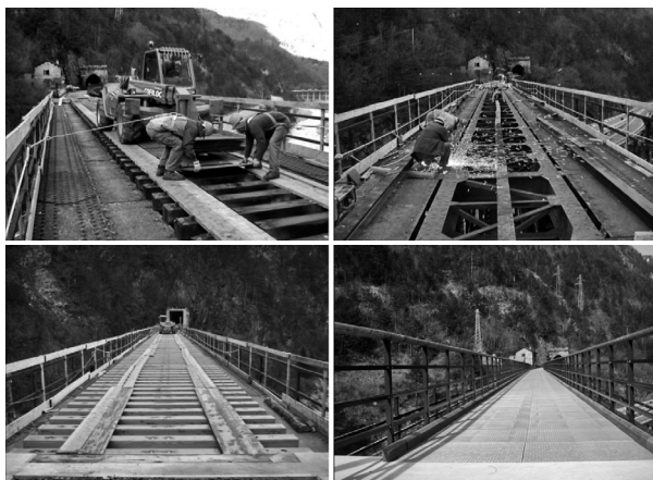
Figure 16. Construction of the new decking. Top, removal of railway sleepers and inspection walkways. Bottom left, the new cross-beams made of glulam larch-wood. Bottom right, the finished decking. As shown by the photographs, employees wore safety harnesses attached via a shock absorber to the life lines at the sides.
